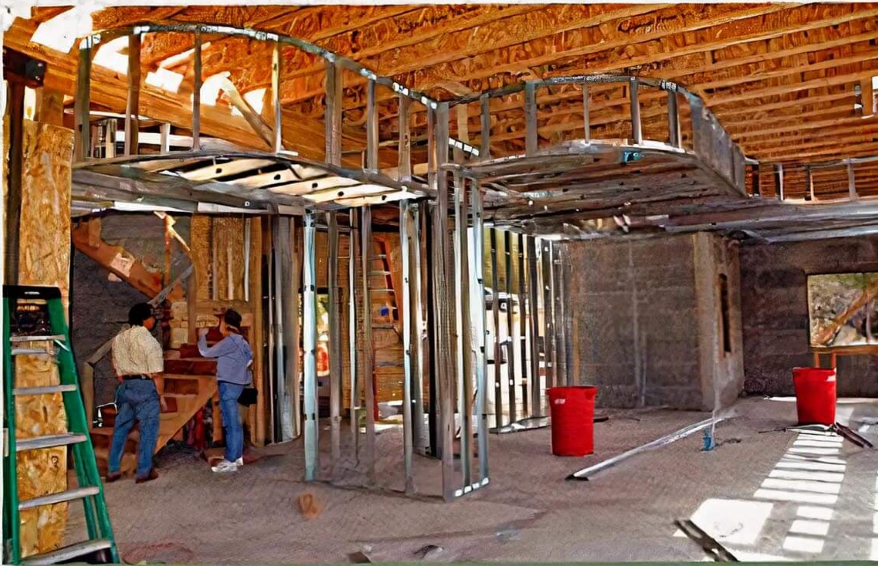
Architect Paul Cate discusses construction progress with homeowner Claudine Mohney.
